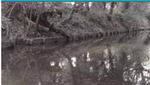
toe-boarded banks, Beverley Brook, Wimbledon Common
