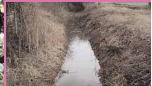
ditch restoration at Crayford Marshes
