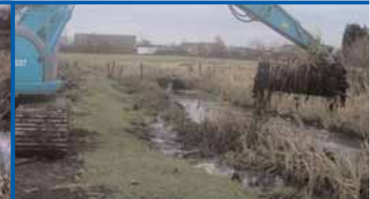
dredging the central channel
