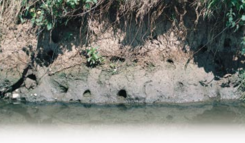
Photo Aquila Photographics
